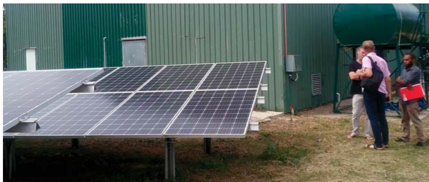
Solar power facilities at Iririki Island Resort
